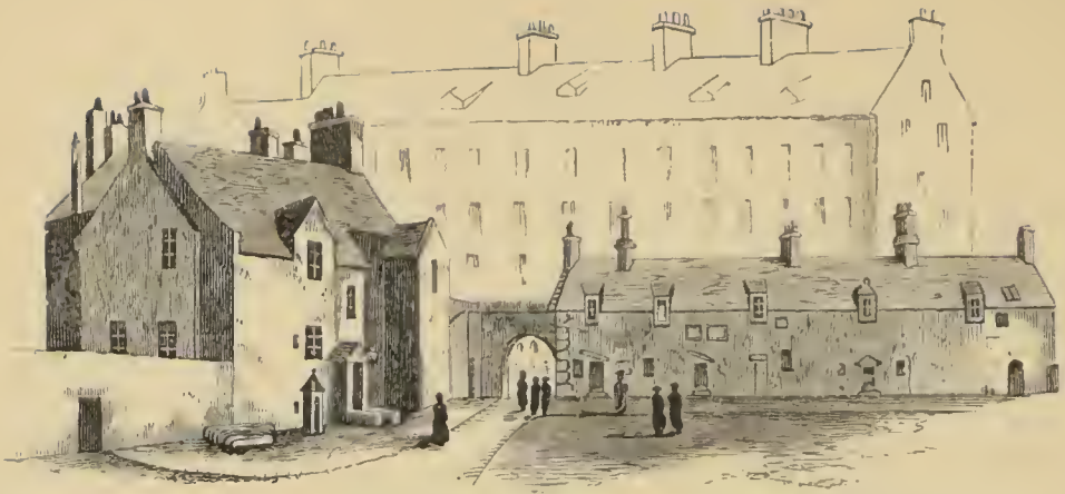
PRINCIPAL ROBERTSON'S HOUSE, WITH THE GUARD-HALL AND TEVIOT CHAMBERS (1789).
